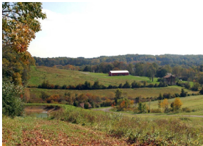
Pole Barn removed, land recontoured to create overlook gathering spaces.
